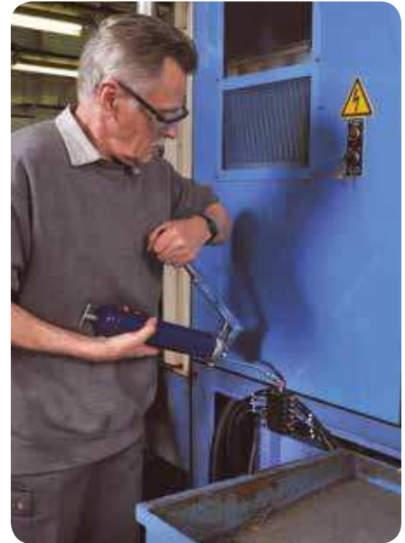
This single-point metering valve enables this technician to lubricate ten bearings without removing any guards or shutting down the production line.
